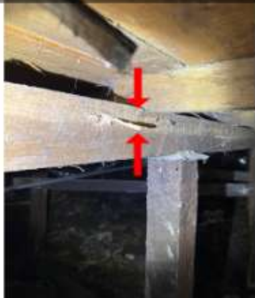
Half of timber bearer damaged by wood borer attack
