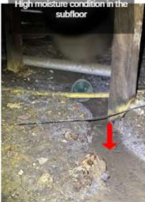
Suspected leaky service pipes under subfloor
