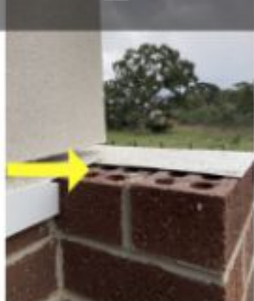
Missing flashing with water entry in to brick wall
