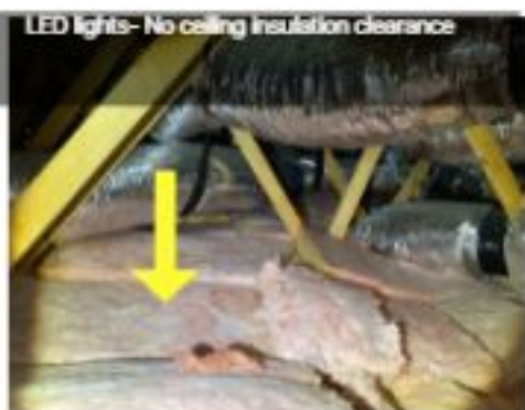
FIGURE 4.7 DEFAULT MINIMUM CLEARANCES FOR RECESSED LUMINAIRES
