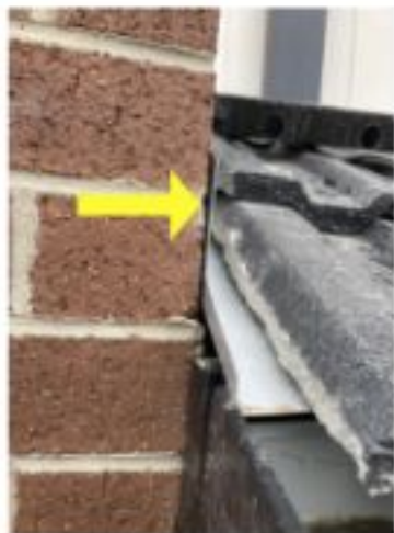
Missing flashing with water entry in to brick wall
